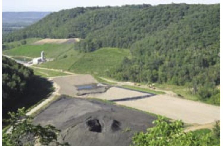
Dairyland owns and operates the Alma Offsite near its Alma, Wis., power plant site. The Genoa facility would include a truck maintenance shop, pond for stormwater management, heavy equipment for material handling and an on-site domestic well and wastewater treatment system.
