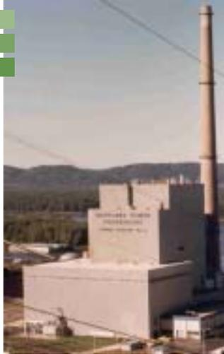
The efficiency of any coal-burning station is measured by the amount of electric energy derived from the amount of fuel consumed. G-3 is extremely efficient, due mainly to a unique double reheat of the steam and super critical steam pressures.
